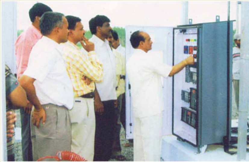
Inauguration of New 33/11 KV Sub-Station at Ramakrishnapur, Adilabad District on 27-09-09 by Sri Ch. Narasimha Reddy CMD, APNPDCL
